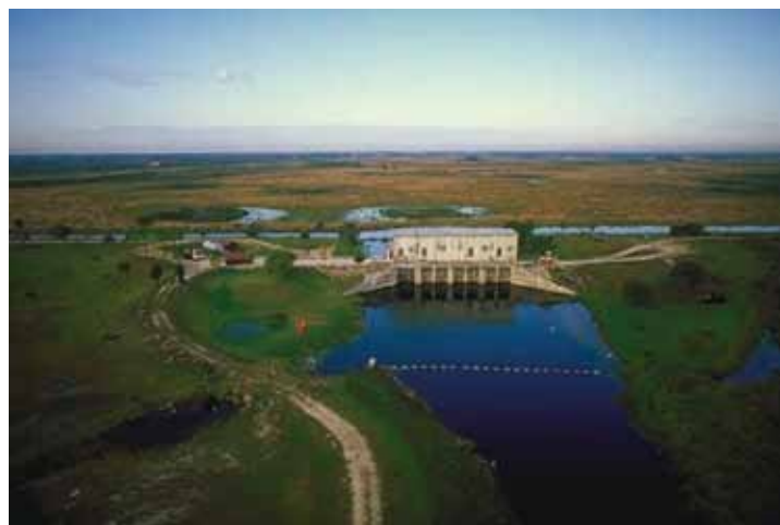
The S-140 pumping station. (South Florida Water Management District)
